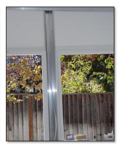
The electrical utility mullions (vertical channel between modules) allows for both interior and exterior lighting and switches.
