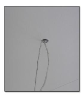
The wiring for the fan beam runs behind the insulated panels in the wall attachment channel. You will want to run the wiring into the fan beams as you install each fan beam panel. The pictures above show how to pull the wiring from within the fan beam after the roof panels have been installed. Be sure to mark you fan beam location on the underside of the roof so you can drill your hole in the center of the fan beam!
