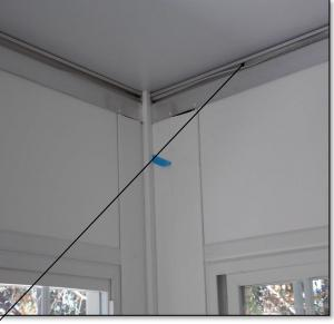
The top wall headers will carry your electrical to your vertical channels between modules created by the electrical mullions. A piece of scrap EPS core material put in the corner will help keep your wiring in place as is turns the corner in the header.
