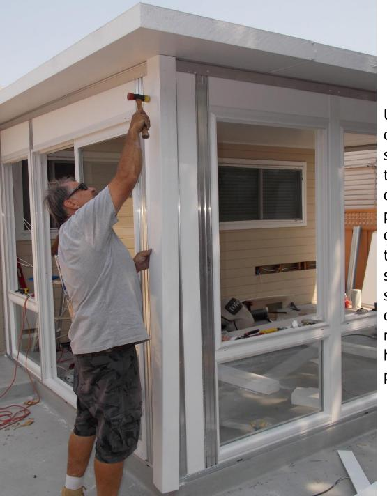
Use a plastic or rubber nonscuff hammer to tap the cladding onto place. Snap on one side at a time and stretch the second side over the snap rib and hammer into place.
