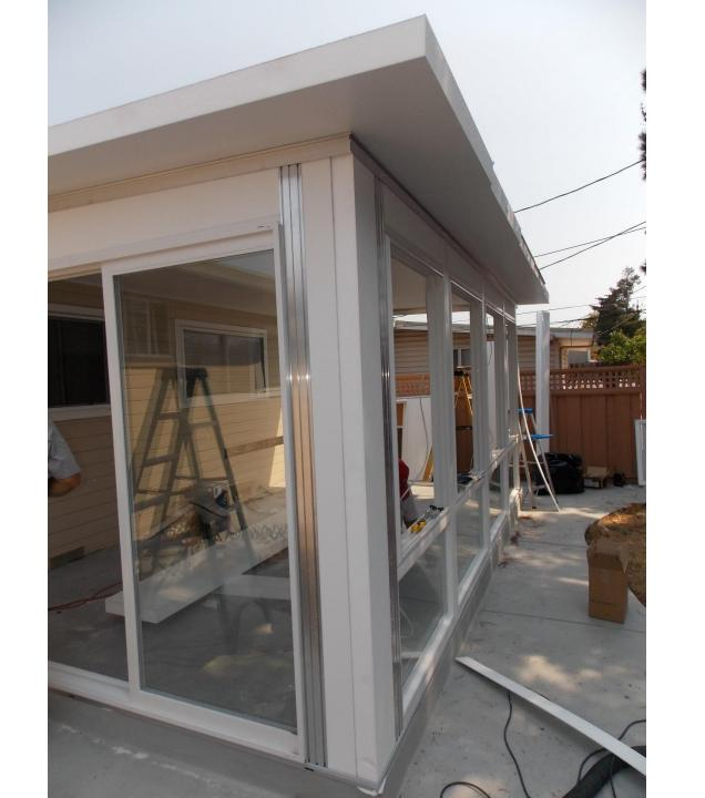
Measure and cut the aluminum corner piece the same way as the wall panel. So that it will slide up into the header channel and then down into the floor channel. Remove all the "Ribs" on each side of the corner piece about 2" from both ends. This allows the corner to slide into the header and floor channels.
