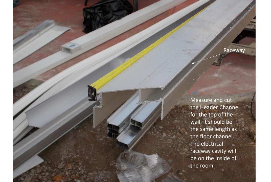
If your modules are plumb, you can measure the distance from the last module to the side wall at the bottom and the measurement for the header channel will be the same.
