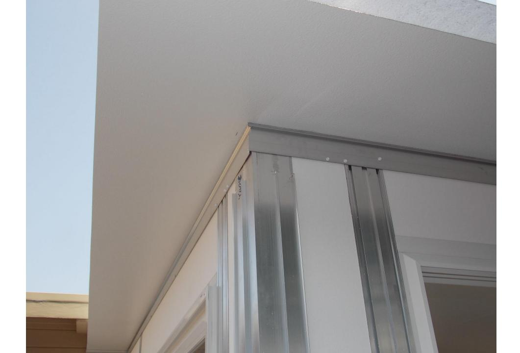
Measure and cut the Vinyl corner cladding to fit.
