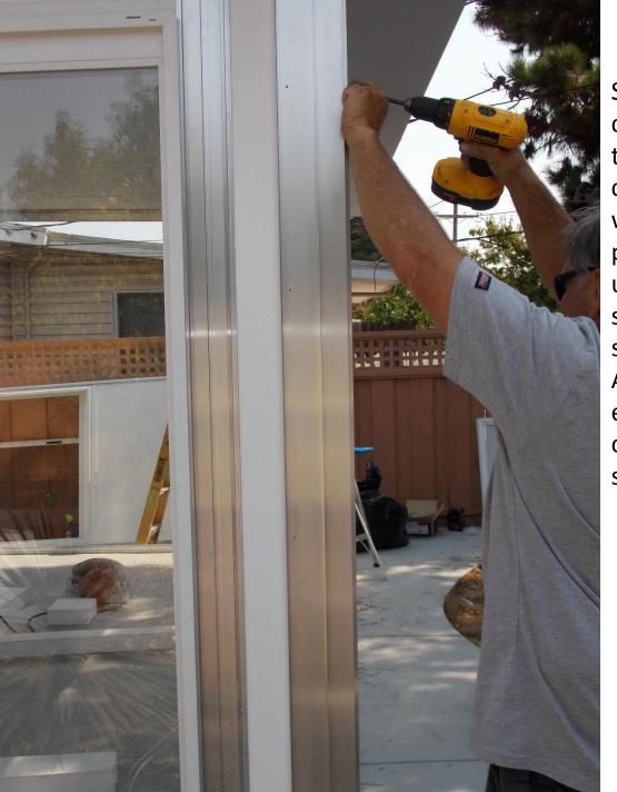
Screw the corner to the corner wall panels using the screws shown. About every 16" on both sides.
