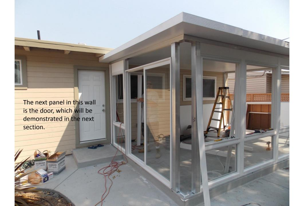
Once you have installed the last module of the wall, you will measure and cut the wall panel to fit into the corner. Once again, the header channel is deeper than the floor channel so you can slide the wall panel up and over the floor channel and then down into the floor channel. Secure into place with a screw as show previously.
