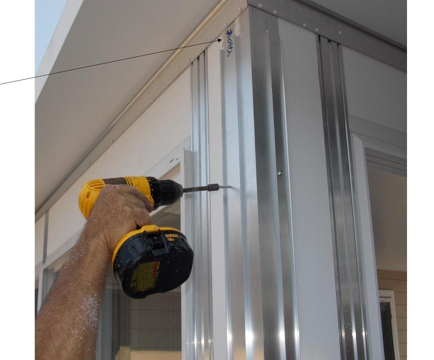
Screw the corner to the header channel and to the floor channel
