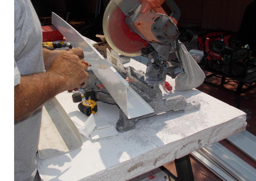
Notch the vinyl cladding enough to fit over the floor channel and the header channel. Each side and each end.
