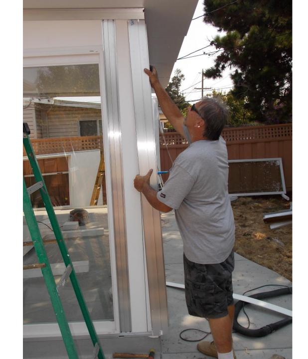
One side of the corner piece is wider than the other. The wider section covers the exposed edge of the corner wall panel.
