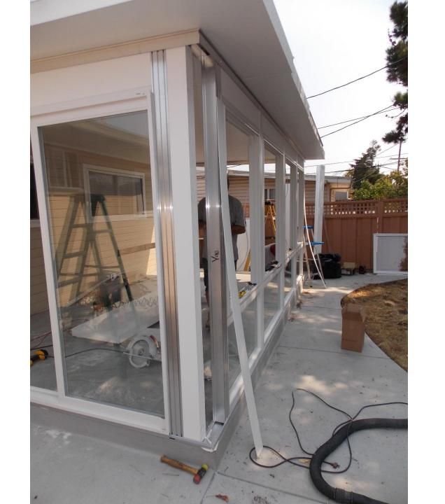
Measure and install the wall panel for the front wall as shown
