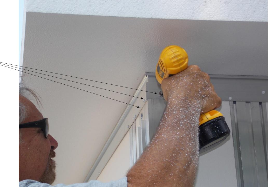
Screw the corner to the floor channel just like all the modules are screwed to the floor channel
