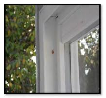
Install the sliding door rail inside the track of the door. Weep holes to the outside as shown. Tap firmly into place with a block of wood and hammer.
