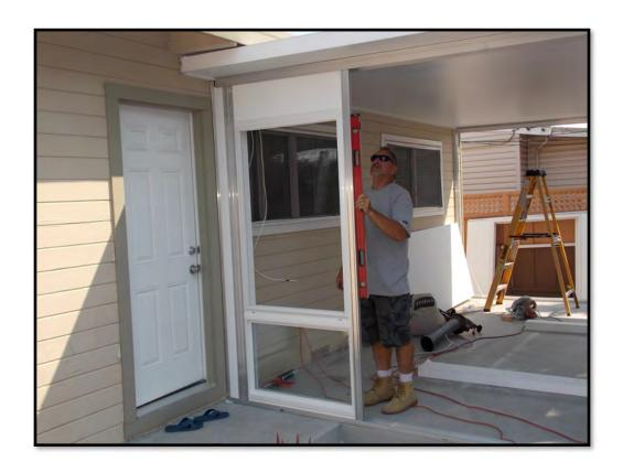
This "H" piece is placed in the floor channel and can be used for leveling the door as needed. It is pre-cut to size. *Please note, this step is not needed if the slab is level.*
