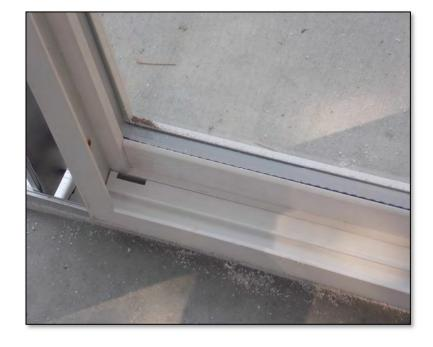
This is the threshold filler piece. It does have an inside and outside, make sure you have it the right direction and cut to fit and notch as shown. It goes between the fixed door panel and the side of the door. Tap into place.
