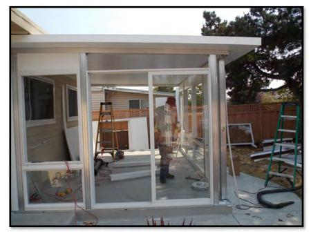
The vinyl "H" piece rests on top of the door and receives the wall panel after it is cut to size. Lay it on top of the door so you can get the correct measurements for the solid panel. It is already cut to size.
