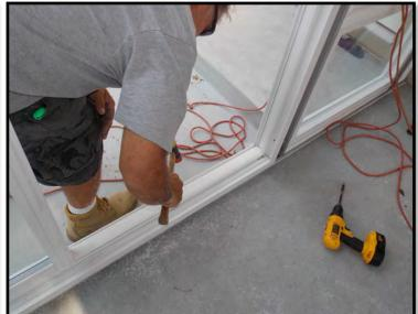
The sliding door panel is lifted into place by inserting the top of the door in first and sliding the bottom of the door over the threshold. Rollers, of course to the bottom.
