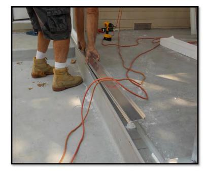
For leveling the "H," you can secure it into place using a few set screws inserted through the floor channel.
